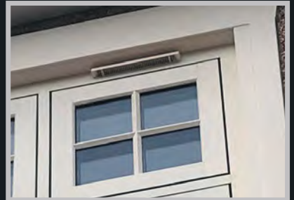
Trickle vent through the Flush Sash outer frame
