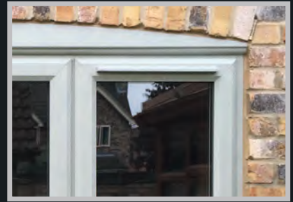
Trickle vent through a Rebated Sash
